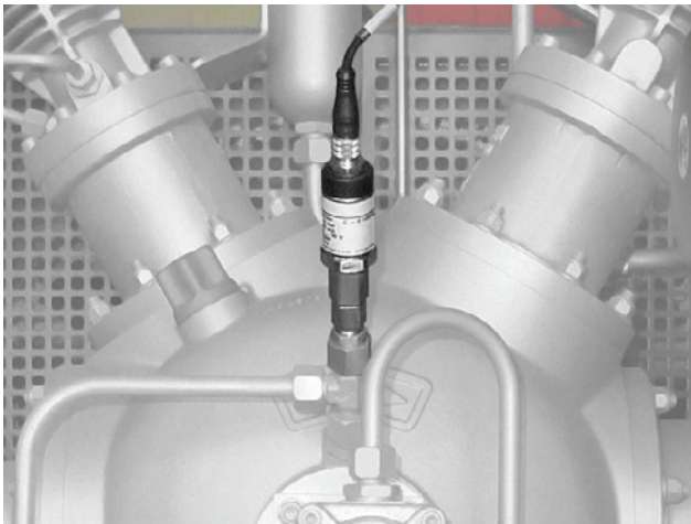
Oil pressure sensor
